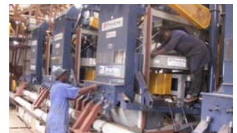
Engineers working at KCU coffee processing plant, Bukop
